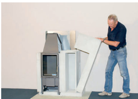
Just follow the supplied guide and assemble all the parts. Fix them in place with the acrylic glue. (4 + 5)
