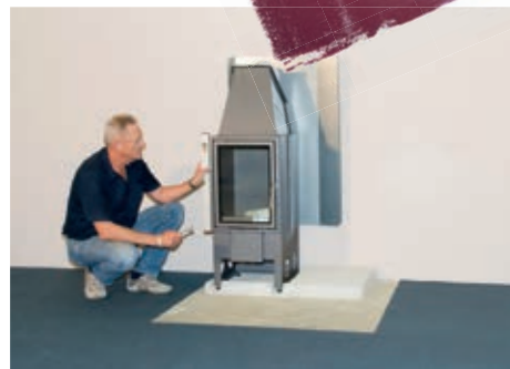
Position the fireplace insert with a spirit level. (3)
