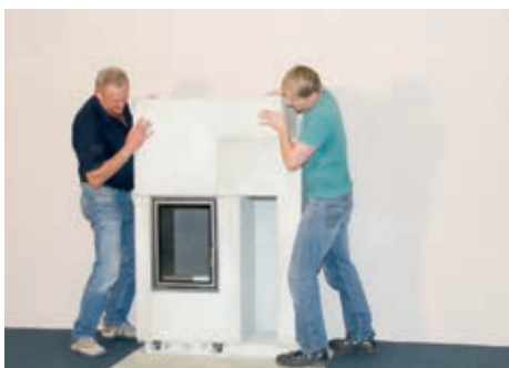
Just follow the supplied guide and assemble all the parts. Fix them in place with the acrylic glue. (4 + 5)
