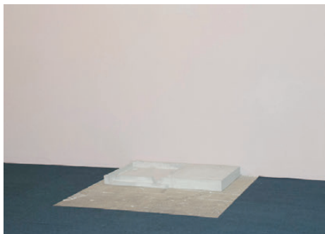
Determine the fireplace location and mark its outline. (1)
