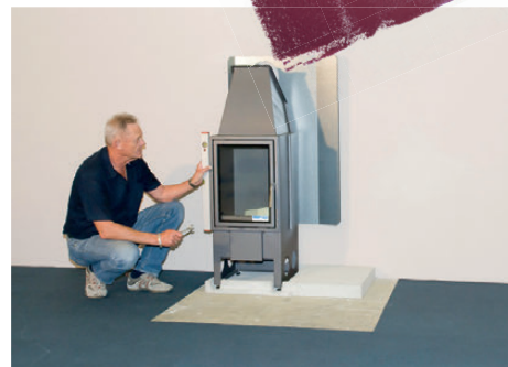
Position the fireplace insert with a spirit level. (3)
